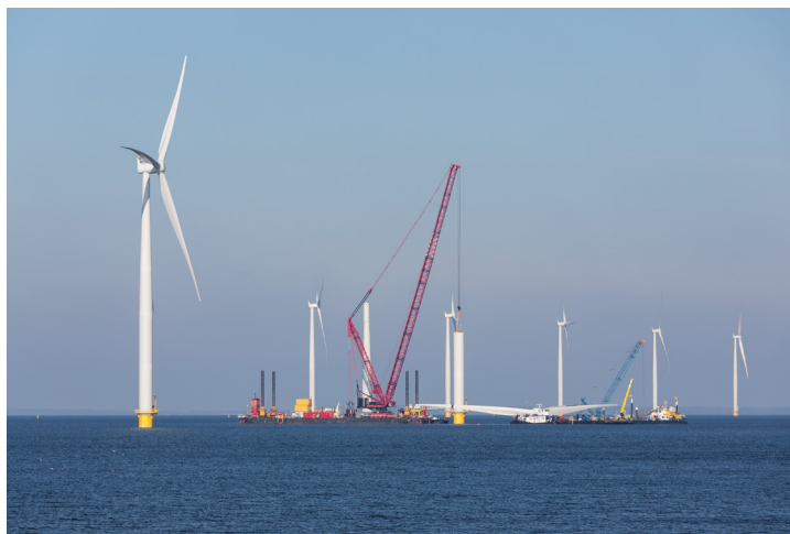
Figure 3: Off-shore wind turbine construction
