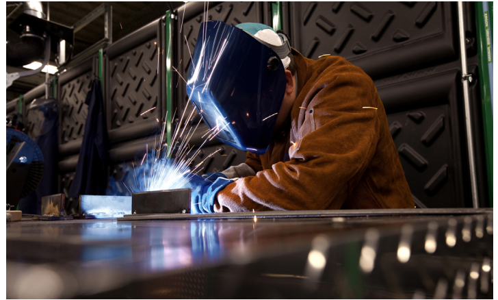
Figure 1. A Linde welder produces fillet welds.
