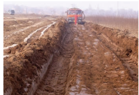
Muddy conditions at a well site
